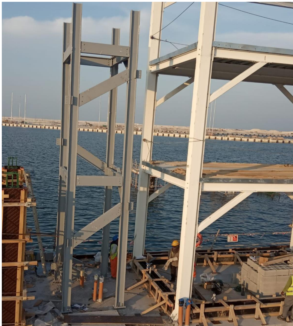
18m Height Control Tower Installation
