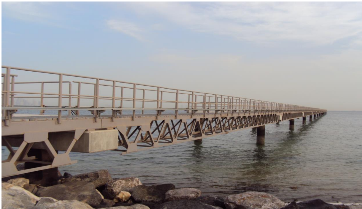
South Side Bridge for Approach Light
