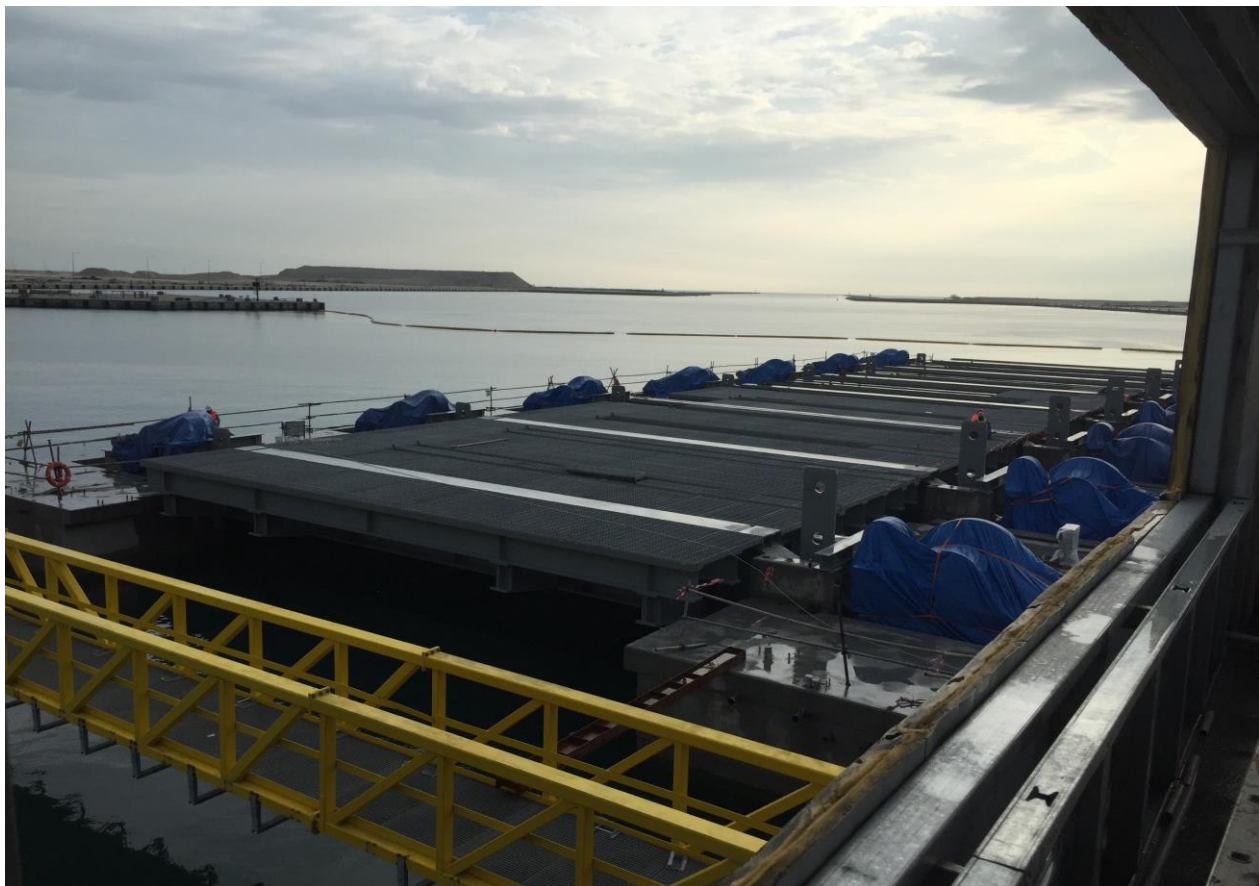
Syncrolift Assembling
