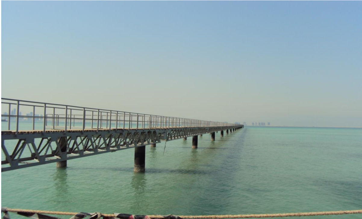
North Side Bridge for Approach Light
